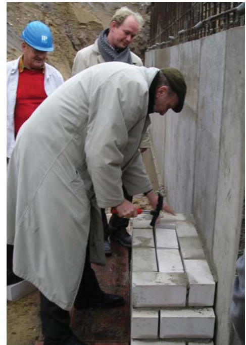
Grundsteinlegung BSH-Labor Laying of foundation stone at BSH laboratory
